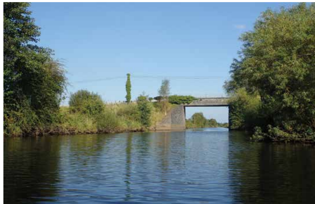
Carrickmakeegan Bridge before arrival at larger loughs.
